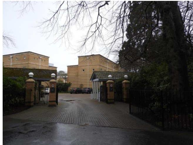
T133, lime. Low branches over entrance.
